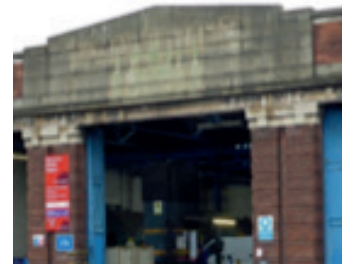
Trent Barton's Manvers Street Depot in Nottingham centre
